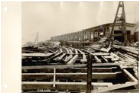
Halifax, N.S.: Railway Pier #4 showing progress of repairs.
