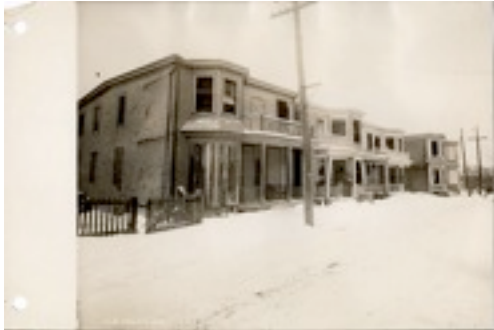
Halifax, N.S.: Damage caused by the explosion.
