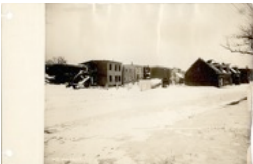
Halifax, N.S.: The damage caused by the force of the explosion over a mile away from the scene of the disaster.
