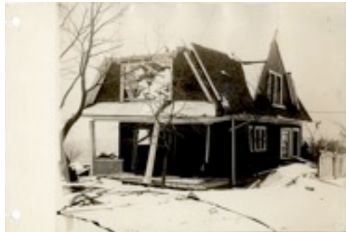
Halifax, N.S.: House. Showing in this case, apparently, the downward force exerted by the explosion.
