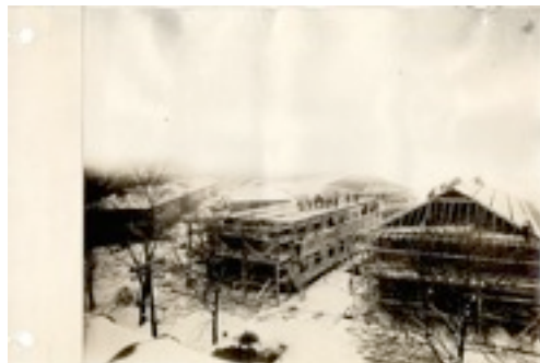
Halifax, N.S.: Administration Buildings for the Halifax Relief Commission at the foot of the Citadel. Photo taken 5 days after work commenced.
