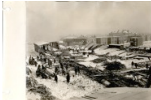
Halifax, N.S.: Another view of the ruins of the car erecting shed at Nova Scotia Works.
