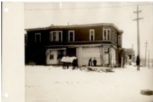
Halifax, N.S.: Damage caused by the explosion.
