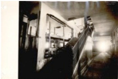
Halifax, N.S.: Interior of Alexander McKay School, showing the destructive force of the explosion.
