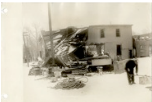
Halifax, N.S.: Damage caused by the explosion.
