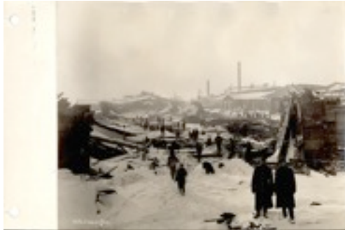
Halifax, N.S.: Ruins of car erecting shed.
