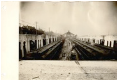
Halifax, N.S.: Interior of the C.G.R. Shop. (more likely, the North Street Station).
