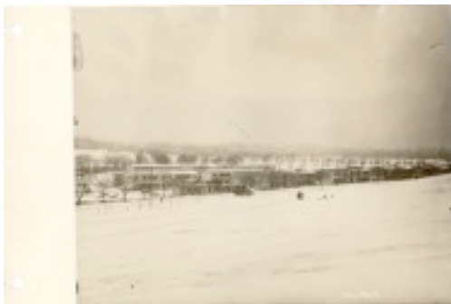
Halifax, N.S.: View of progress of construction on South Common.
