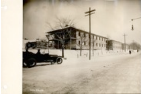
Halifax, N.S.: Apartment Houses. (Military Type) These buildings are 96 feet long, 46 feet wide and 2 stories high. They contain 16 Apartments each. View from Bell Road.
