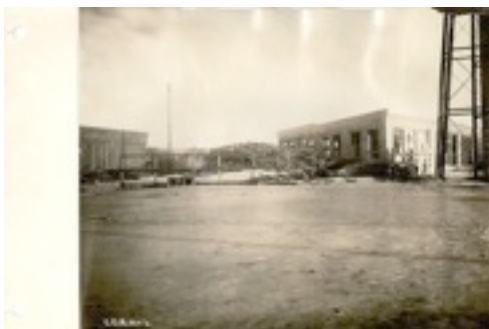
Halifax, N.S.: Exterior of Round House about a mile from the scene of the disaster.
