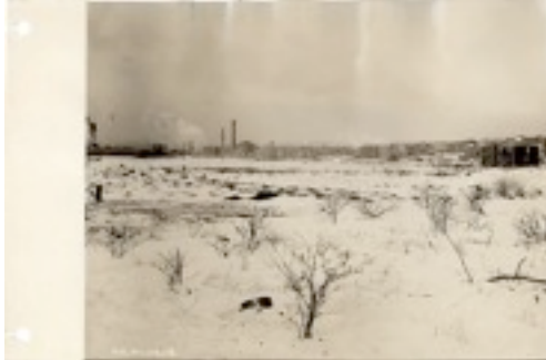
Halifax, N.S.: Damage caused by the explosion.
