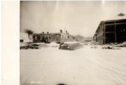
Halifax, N.S.: Apartment Houses. (Military Type) These buildings are 96 feet long, 46 feet wide and 2 stories high. They contain 16 Apartments each. View from Bell Road.
