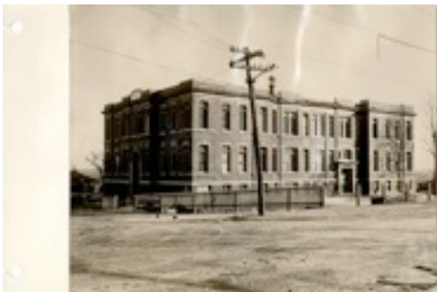
Halifax, N.S.: The Alexander McKay School; a brick and concrete building which had just been completed. The interior of this building was badly wrecked. Now used as a boarding house, and with a wooden addition at the back accommodating over 1800 men.
