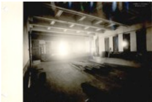
Halifax, N.S.: Interior of Alexander McKay School, showing the destructive force of the explosion.
