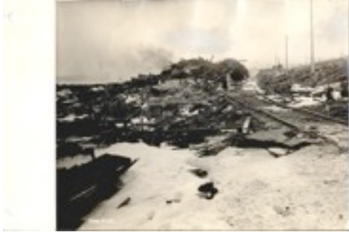
Halifax, N.S.: Ruins of the Sugar Refinery. A ten story building.
