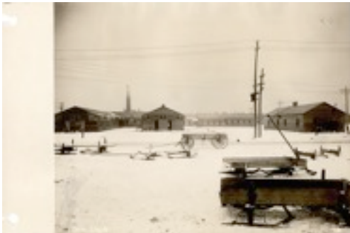
Halifax, N.S.: Temporary housing for workmen of contractor, clearing up devastated area.
