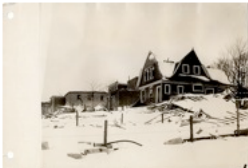
Halifax, N.S.: Damage caused by the explosion.
